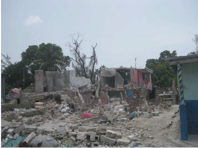
Fig. 9: Even five months after the earthquake, rubble blocks and slows travel on roads in many parts of Port-au-Prince, leading to horrific traffic congestion and continuing to make sections of the city impassable. Rubble removal is the first critical step towards reconstruction; it is a precursor to accessible roads, ports, airports, as well as improved infrastructure such as water, sewage and electrical systems. Until the rubble is removed, Haitians will not be able to return to their pre-earthquake communities. June 8, 2010
